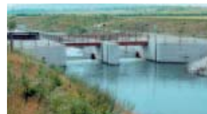
Wehr 3 in Gerasdorf
